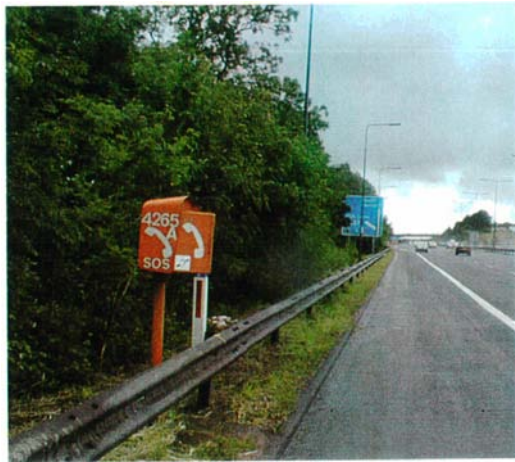
327 telephones at strategic locations along 135km of motorway
