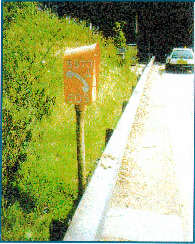
Existing Emergency Roadside Telephone
